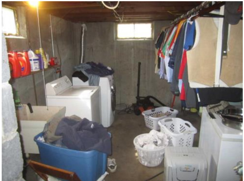
36 Dwelling/Basement/Laundry Room - Laundry Room (1) Date Taken: 8/14/2014 Taken By: Tom Balmes North
